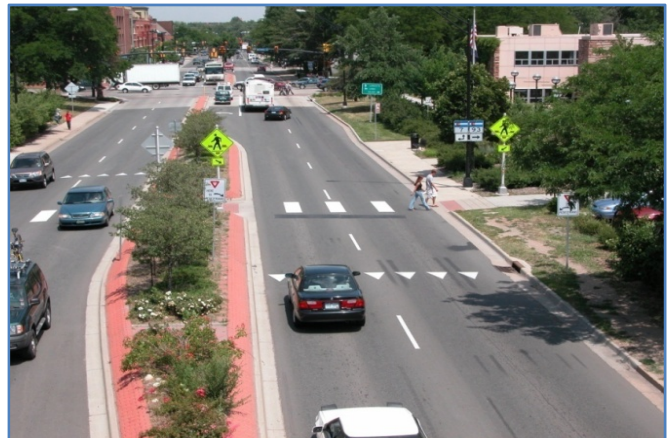
Example of pedestrian refuge islands with pedestrian actuated signals that stop traffic only when a user is present, visible crosswalks, and appropriate signing.
