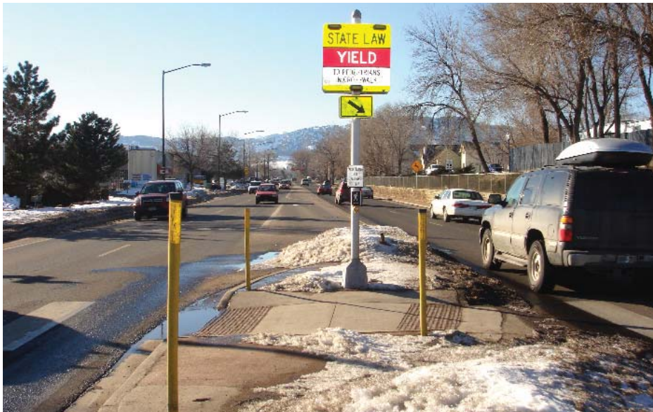
Examples of pedestrian refuge islands with pedestrian actuated signals that stop traffic only when a user is present, visible crosswalks, and appropriate signing.
