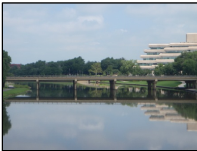
1 st Street Bridge
