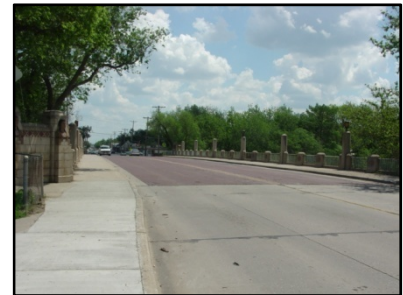
Bridge with Sidewalks
