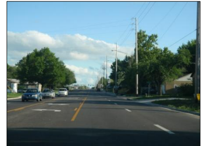
Recently Completed Project on Oliver
