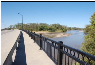
83 rd Street S. Bridge Over Arkansas River
