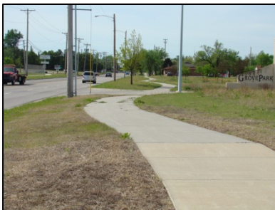
Sidewalk along Hillside Street
