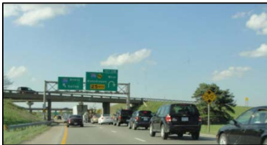
Congestion at I-235 Exit
