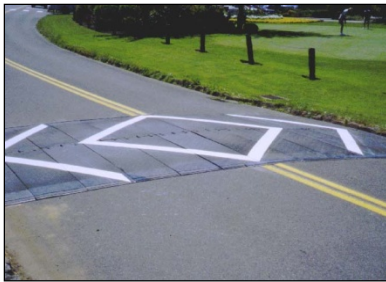
Traffic Calming Example: Raised Pedestrian Crossing
