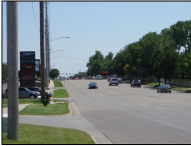
Driveways and Dedicated Left Turn Lane
