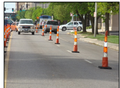
Construction on Broadway
