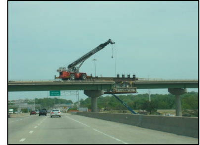
Rehabilitation of a Bridge over US-54/400 (Kellogg)
