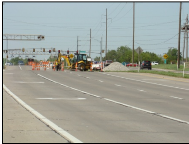
Construction on K-15
