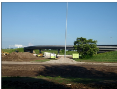
Maintenance on Freeway Ramps
