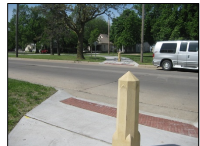
ADA Compliant Curb Cut
