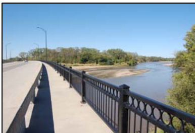
83 rd Street S. Bridge Over the Arkansas River with Bicycle/Pedestrian Crossing
