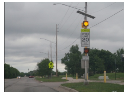
School Zone Warning Signal
