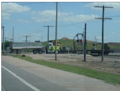
At-Grade Rail Crossing
