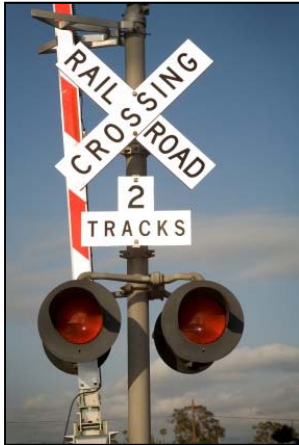
Rail Crossing Safety Features
