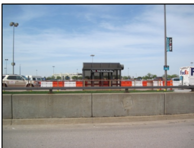
Transit Stop at Mid-Continent Airport
