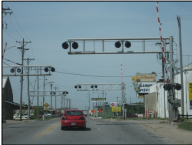
At-Grade Rail Crossings
