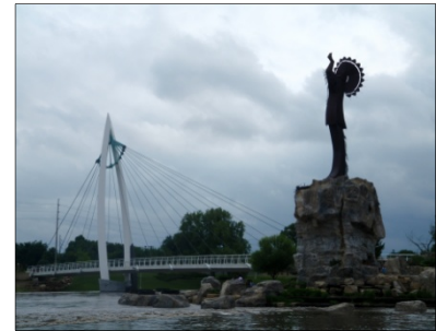
Pedestrian Bridge at Keeper of the Plains
